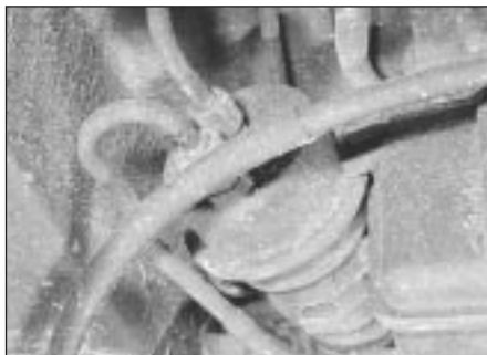
21.1 Fuel accumulator unit location
