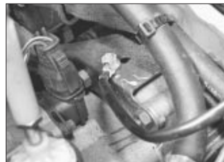
5.8c Earth strap to gearbox
